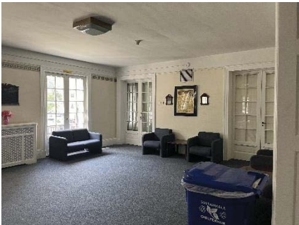
Interior walls and wood trim
