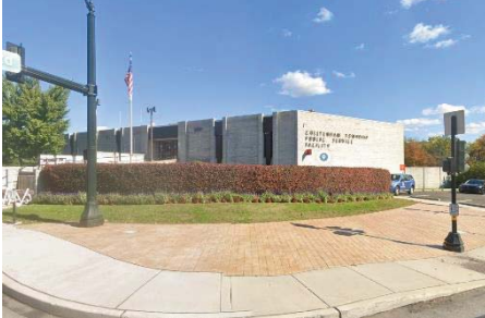
Public Works Building
