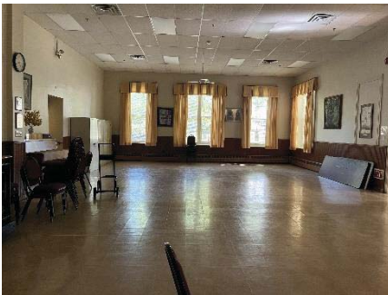
View of main hall flooring
