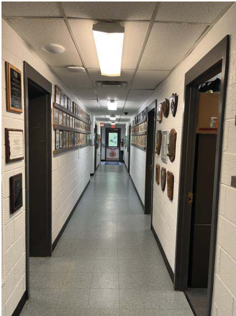
View of VCT flooring and CMU block walls
