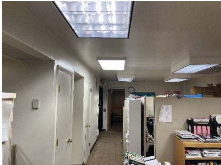
Suspended plaster ceiling with surface mounted lights
