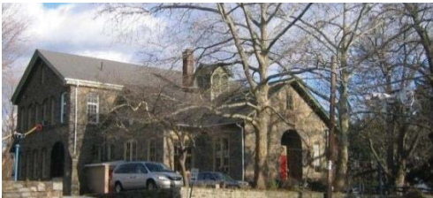
Public Works Facility
