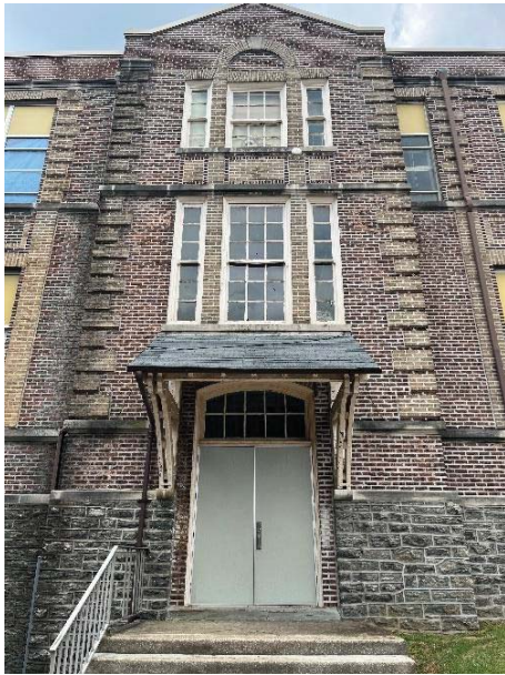
Original School Building
