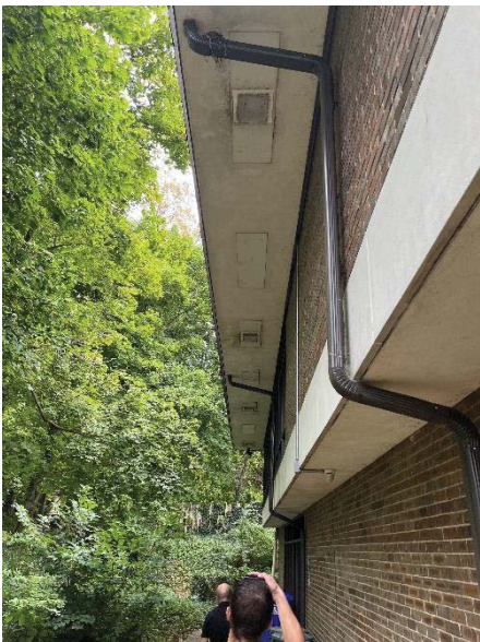
Brick walls at lower level
