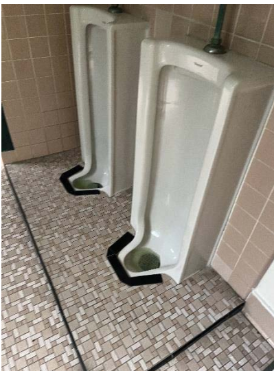
Floor level change at urinals
