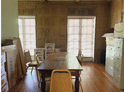
Example of historic wood paneling
