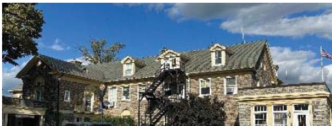
Slate shingles, dormers and flat roof areas
