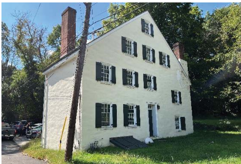
Public Works Facility
