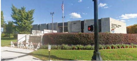
Public Works Facility
