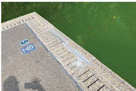
Closeup of coping
