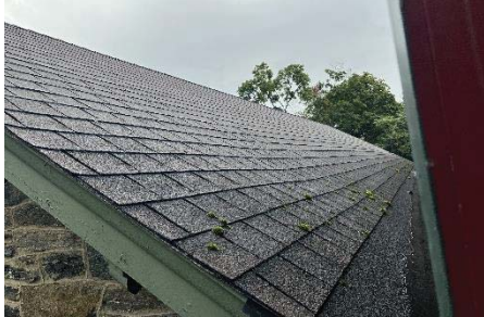
Roof sloping into wall
