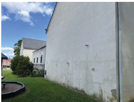
View of stucco wall and roof beyond
