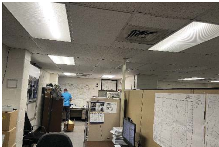
Typical interior ceiling
