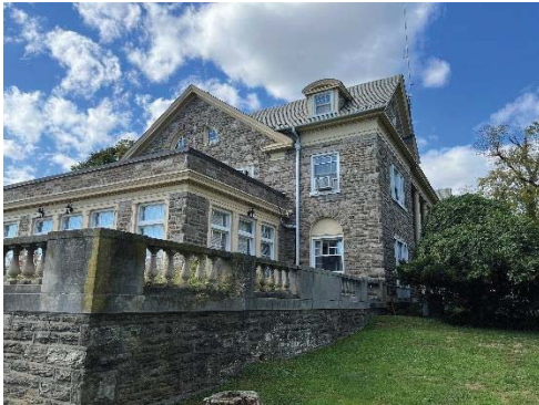
Exterior stone construction
