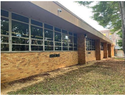
1964 building single pane glass window systems
