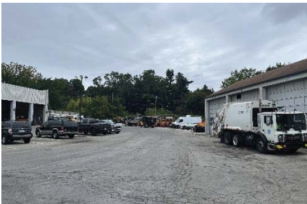
Photo of inner yard with equipment staged along creek
