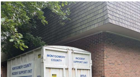
View of Mansard Roof
