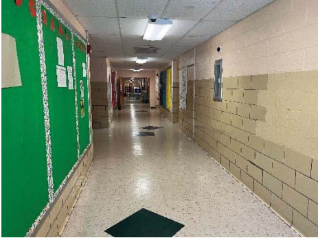
Interior CMU bearing walls in corridor – note glazed block from floor eight course up.
