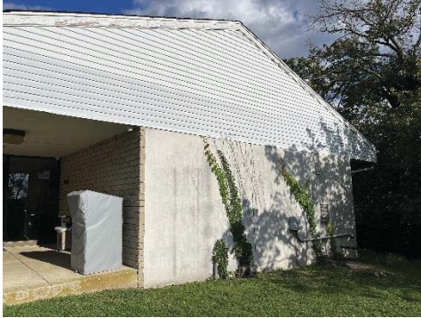
Brick, Stucco and siding
