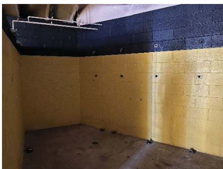
Shower room with all faucets removed for repair
