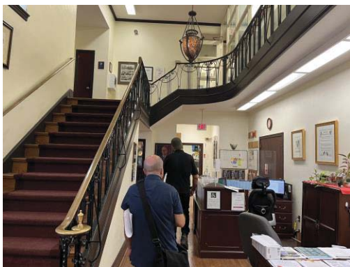
Example of inefficient use of space – reception desk in a corridor, multiple offset floor levels and ornamental stair railings do not meet code
