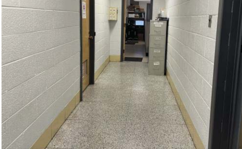
View of Terrazzo Floor
