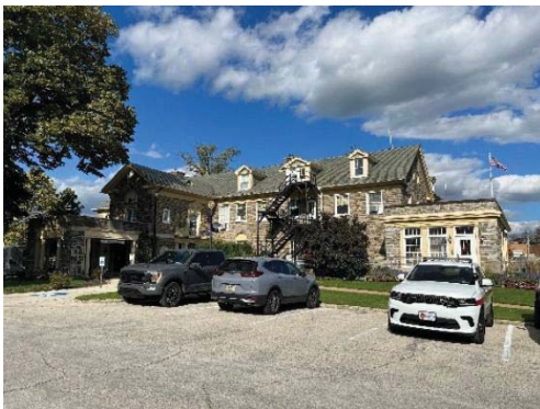
Exterior egress stair
