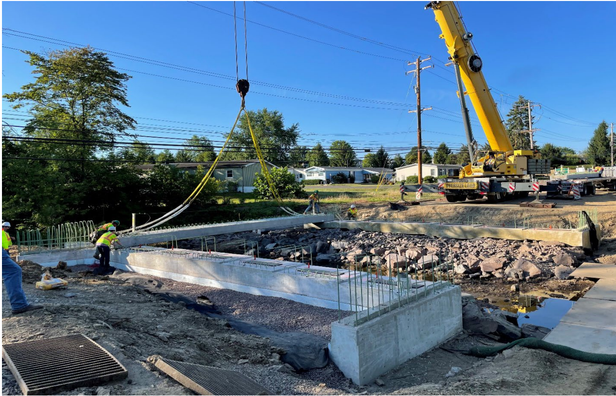
Bridge Beam Setting on Similar Project (Stock Photo)
