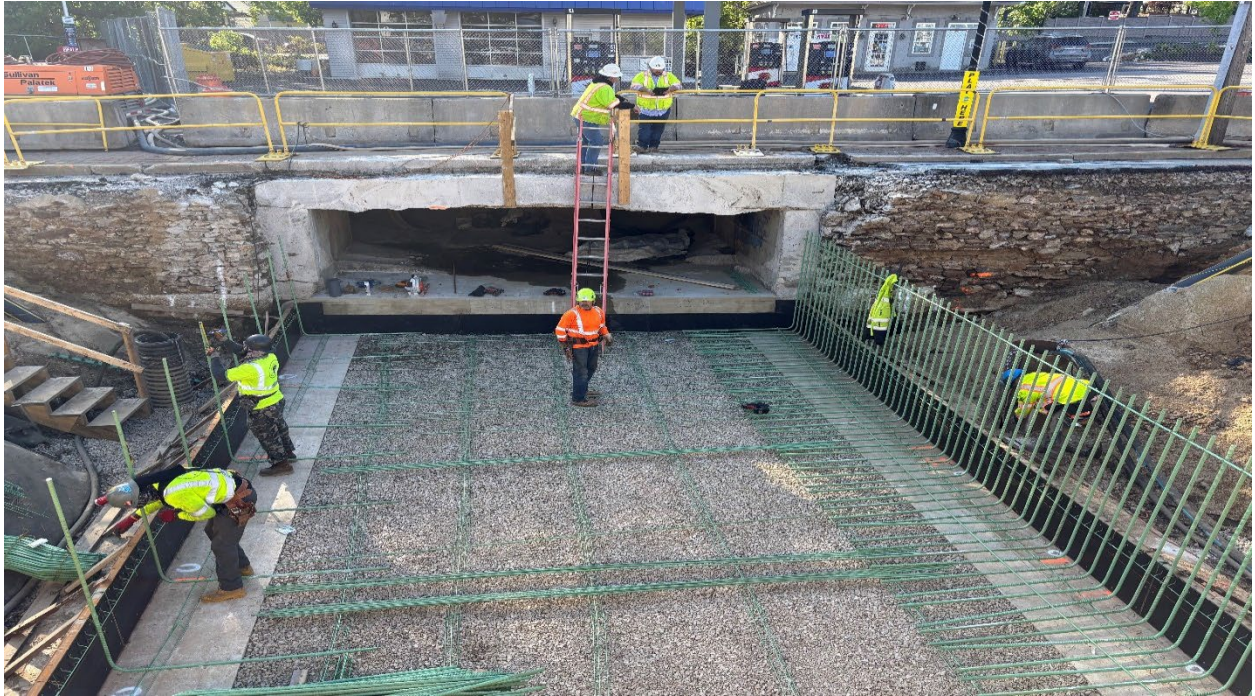
Culvert Floor Preparation – April 2025
