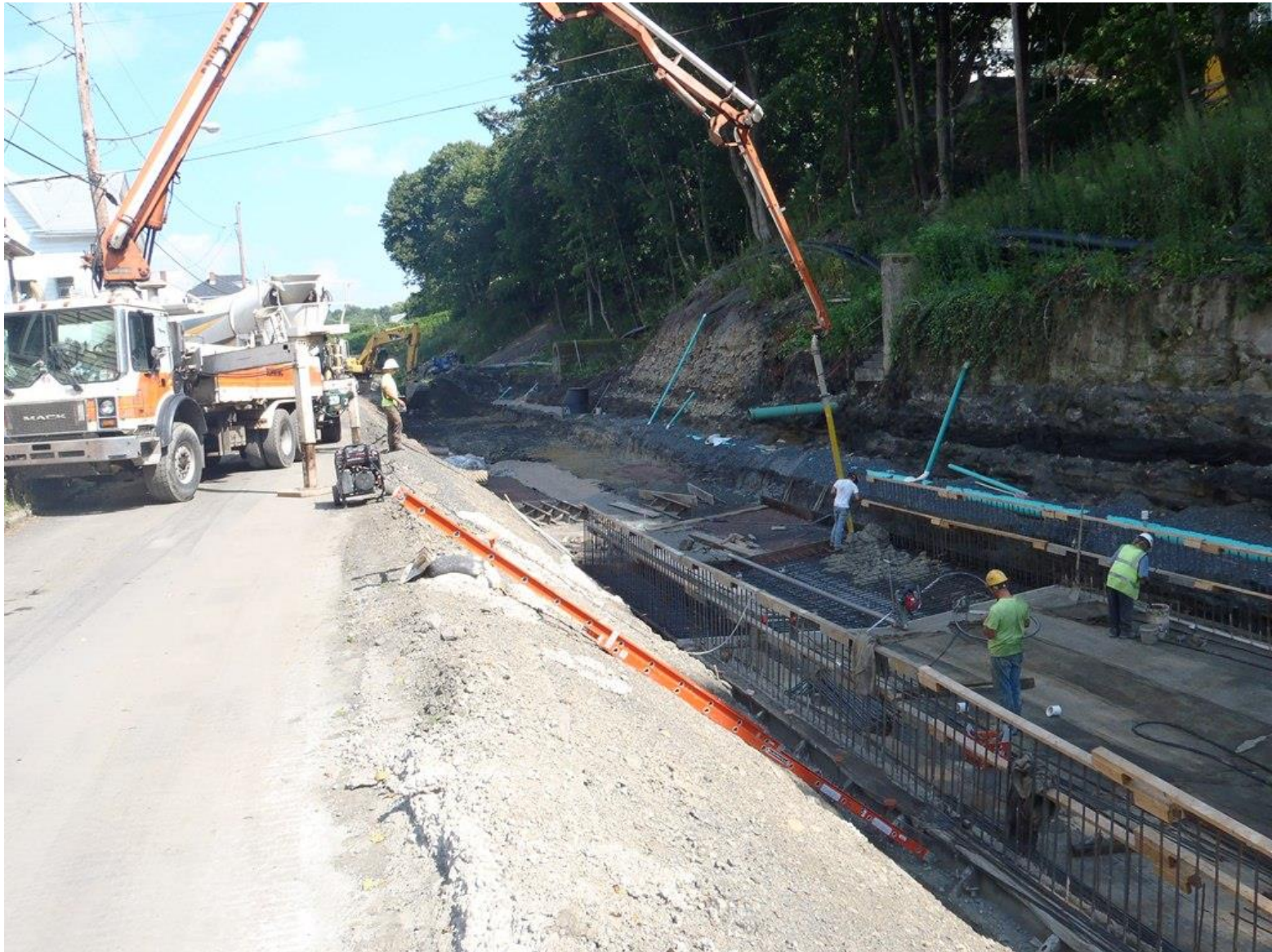
Channel Slab Construction (Shamokin Creek Flood Protection Project)
