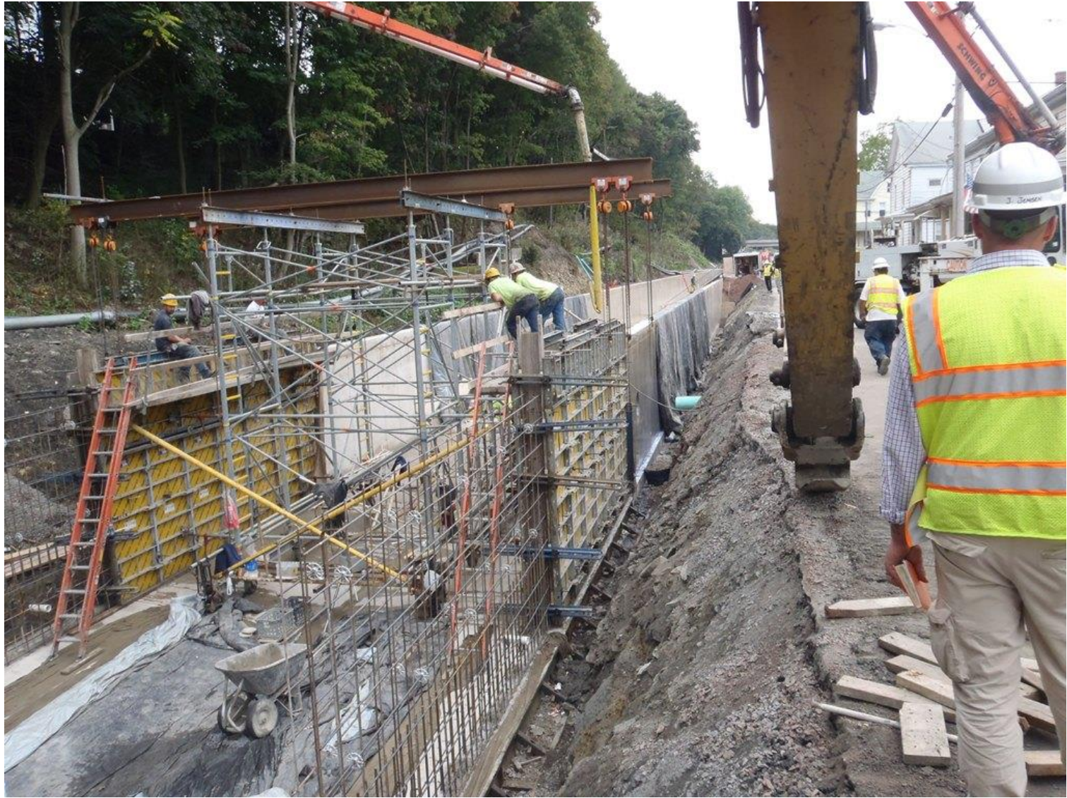
Channel Wall Construction (Shamokin Creek Flood Protection Project)
