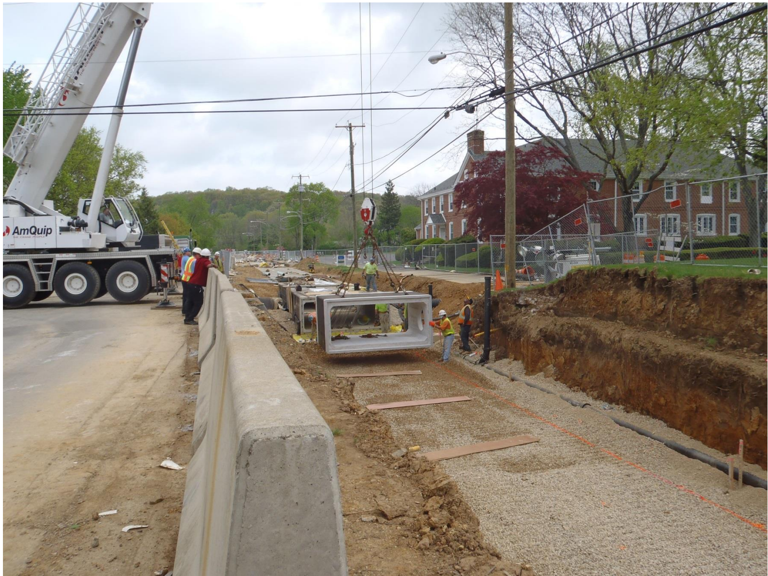
Crane to Set Precast Concrete Box Culvert (Upper Dublin, PA)
